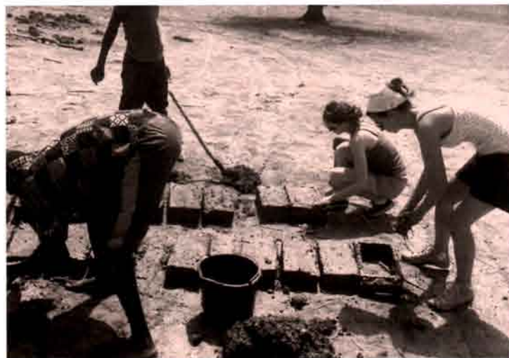
02. FORMING MUD BRICKS IN MOULDS.
